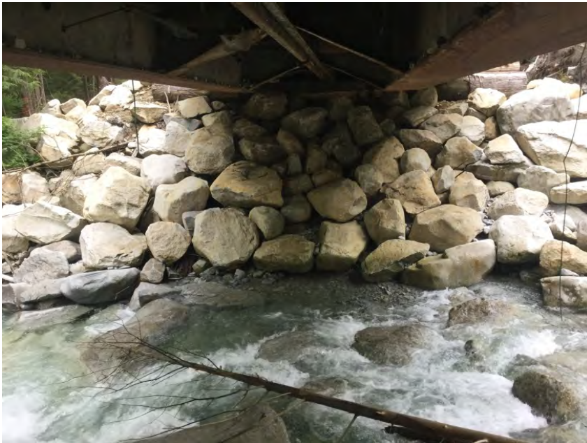
Right Bank Abutment when facing downstream
