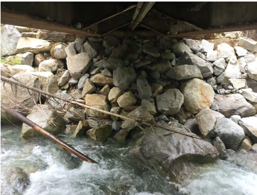
Left Bank Abutment when facing downstream
